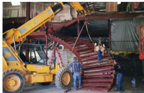
Grand Lobby Staircase Construction
